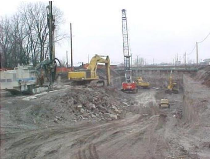
Figure 7: Rock removal operations.
