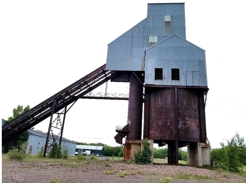
Photograph taken by Linda Harrison of an abandoned hoist
