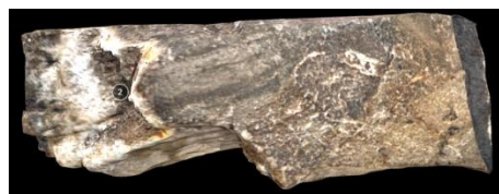
Figure 4. Mackinac Bridge core sample
