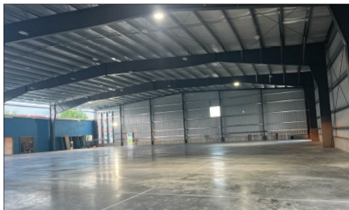
The new MGRRE warehouse space under construction will house Michigan's largest collection of geologic records.
